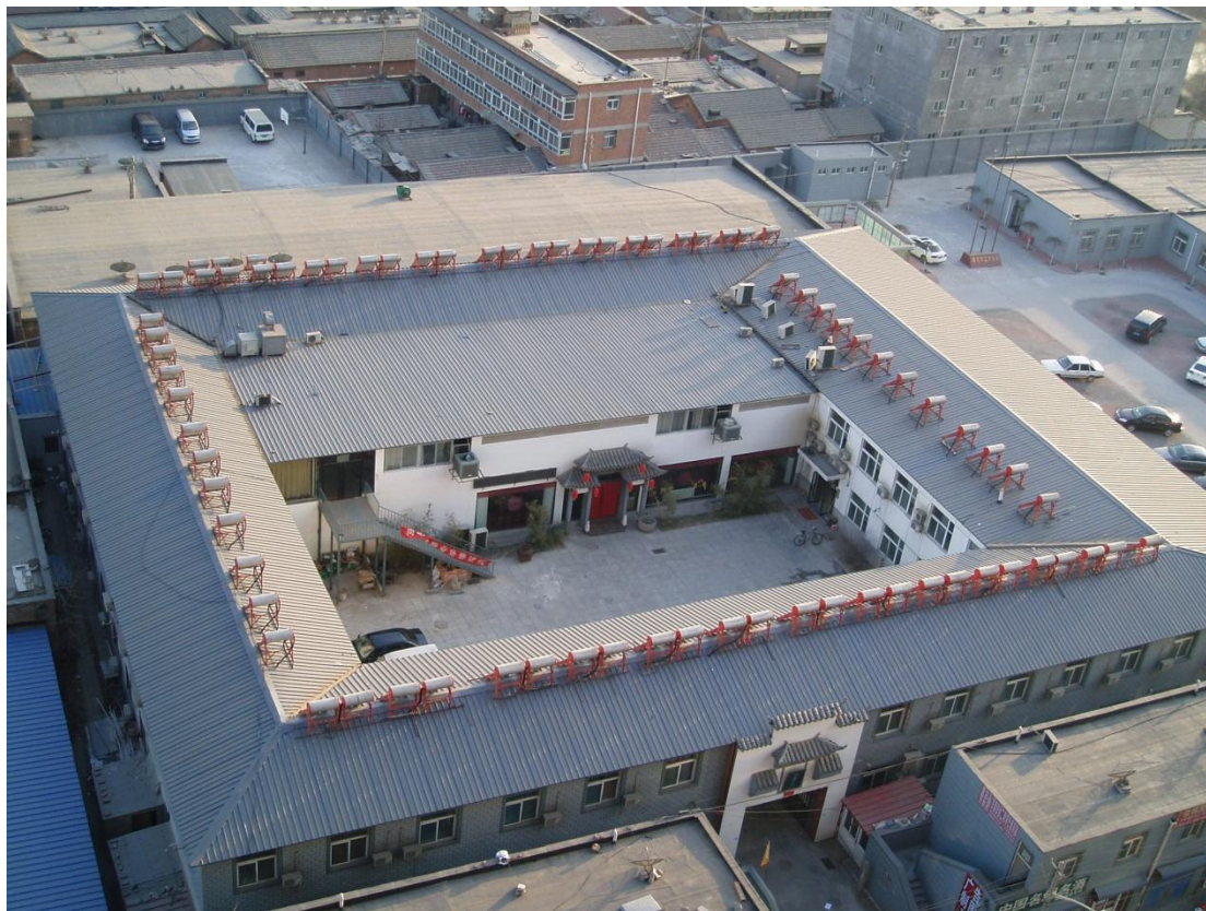
Figure 4: Roof-top installation of solar water heaters in Beijing (photo: first author)
